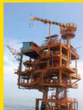
Hydraulic Power Pack
